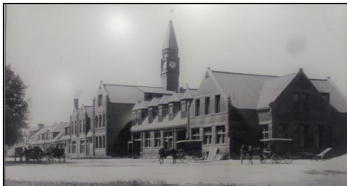
Ogden Railroad Station, 1889-1923
