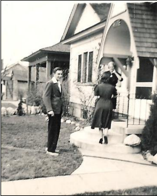
The Krey home about 1940. Note that the triangular porch covering, the railing and the steps are still the same today.
